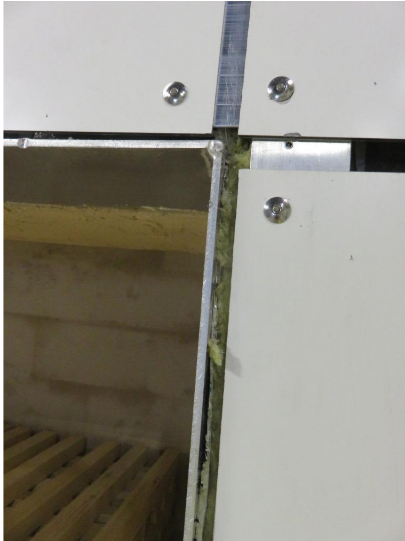
Figure 10. Detail at corner of combustion chamber opening. Panels riveted in place and 20mm vertical gap left for ventilation purposes.
