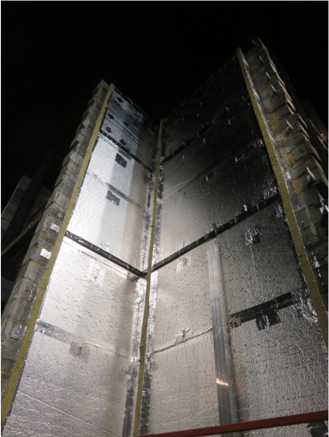
Figure 6. Installed cavity barriers, PIR insulation panels cut to fit and joints taped.
