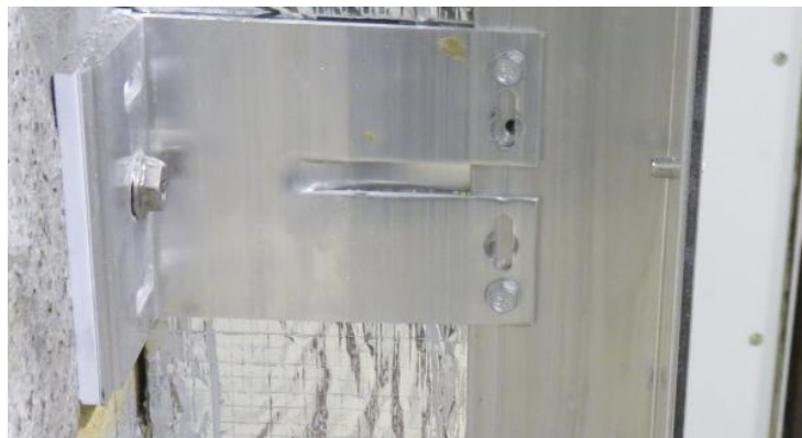
Figure 8. Example of aluminium rail fixed to 'L' bracket through fixed holes.
